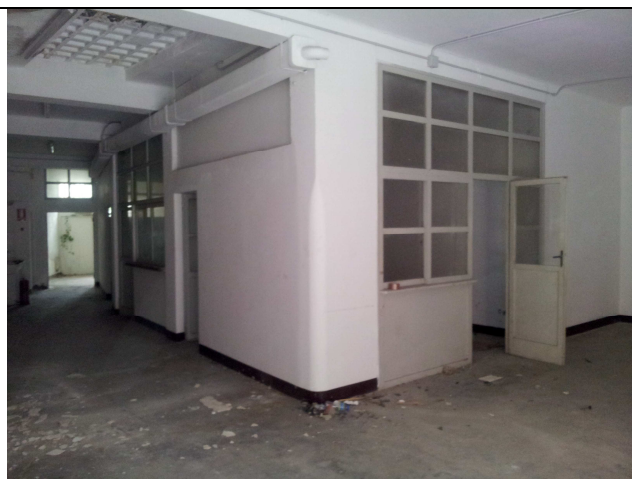
Interni Piano Terra
